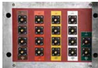
Cam Lock Receptacles with Color Coded Generator Connections
